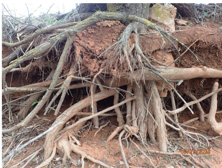
➤ Figure 4. Extensive root systems can provide seepage paths for water.
