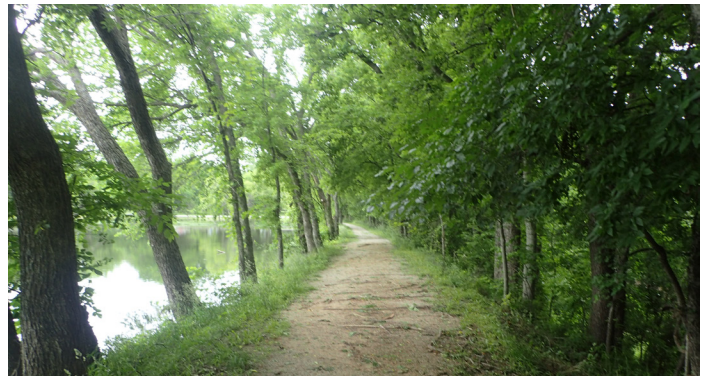
Figure 1. Trees and brush on an embankment limit visibility and can provide a haven for burrowing animals.
