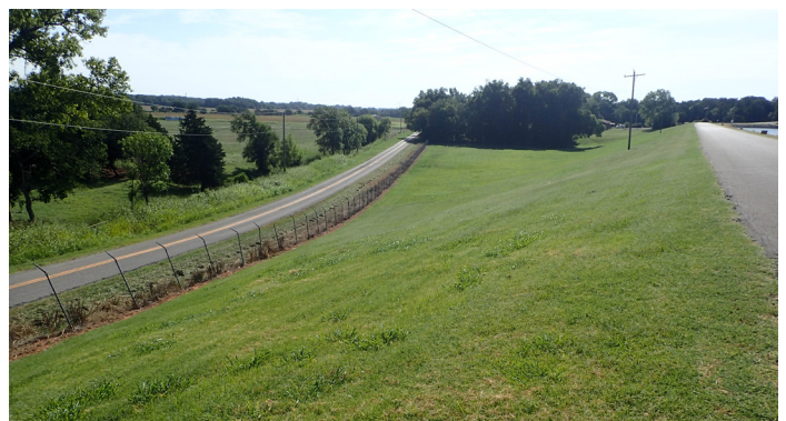
Figure 2. An embankment clear of vegetation and brush with appropriate grass coverage.
