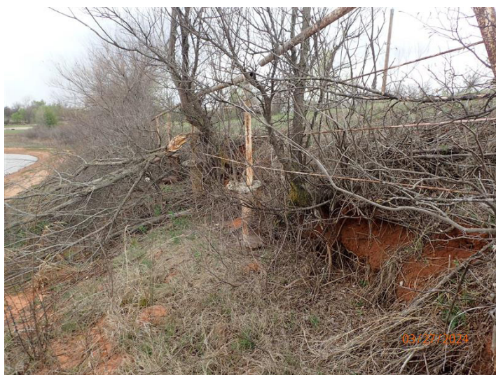
➤ Figure 3. Trees that blow down or fall over can leave large holes that weaken the embankment and increase erosion.
