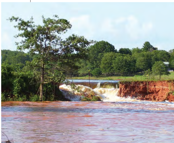
FIGURE 3.1 EMBANKMENT DAM FAILURE IN CLEVELAND COUNTY
