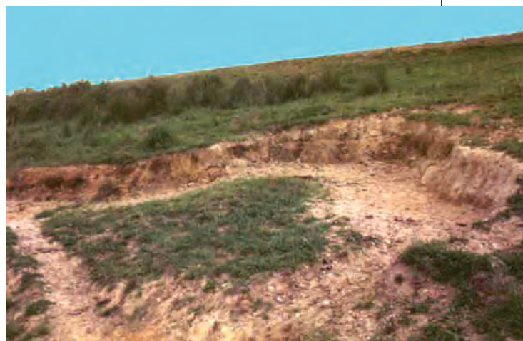
FIGURE 7.1. EROSION OF EMBANKMENT WITH POOR COVER
