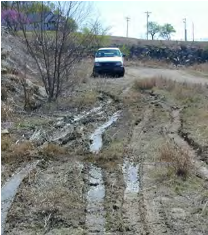
FIGURE 5.5. AREA OF SEEPAGE NEAR TOE OF DAM.
