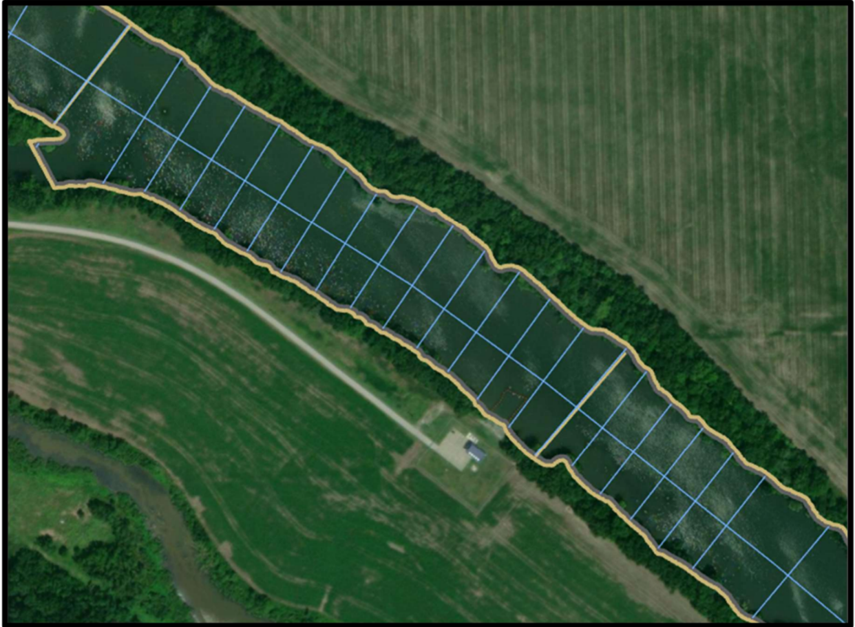
Figure 3. Aerial image of intake showing increased coverage with 100 ft transects.
