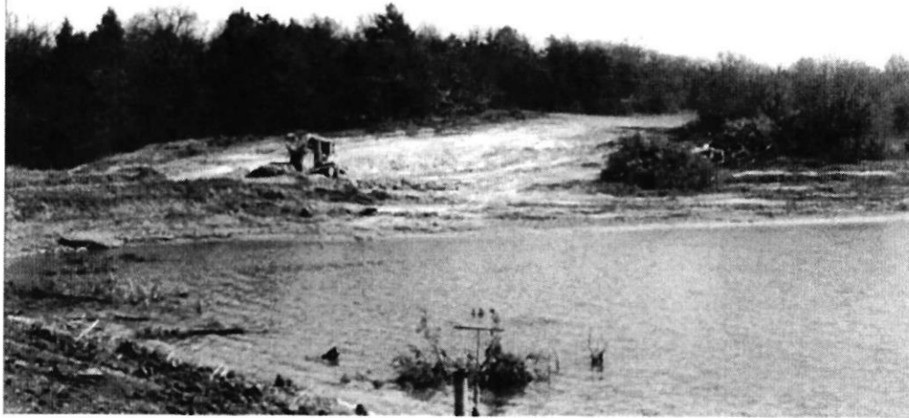
Figure 7. Emergency spillway on the right abutment
