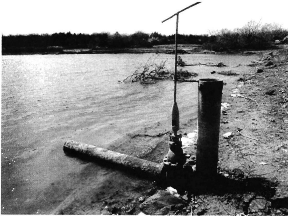
Figure 5. Principal spillway inlet valve
