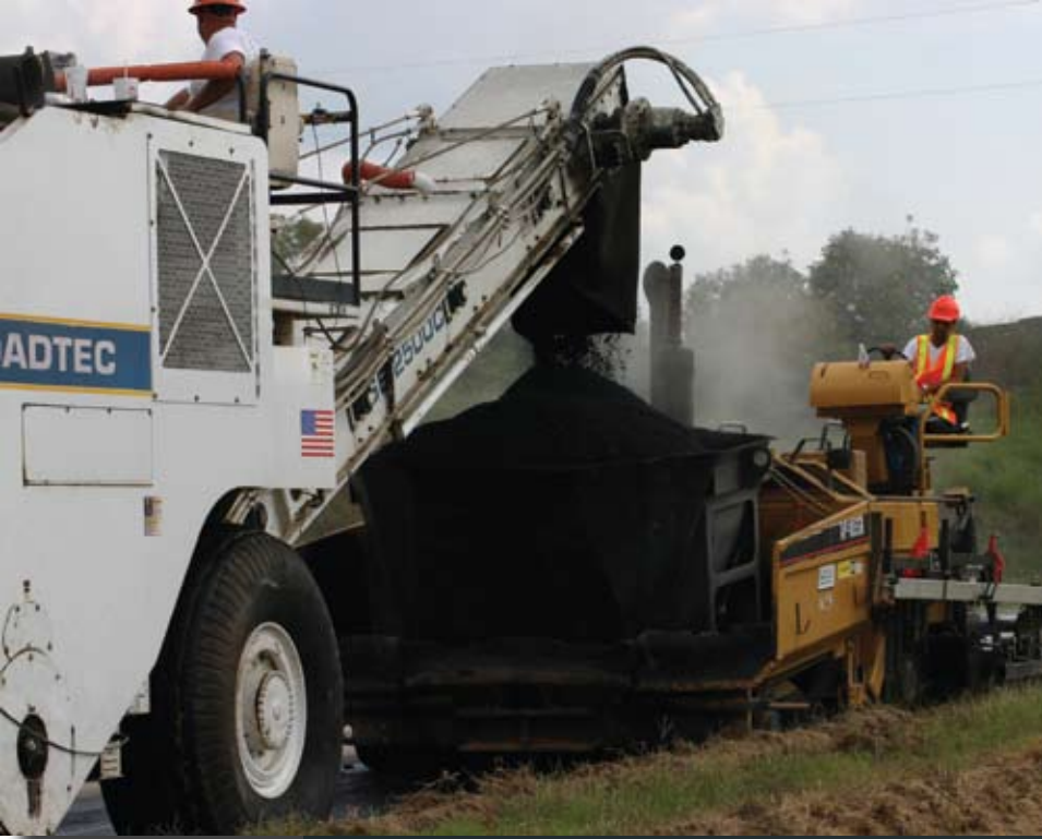
INDIAN NATION TURNPIKE - PAVEMENT REHABILITATION
