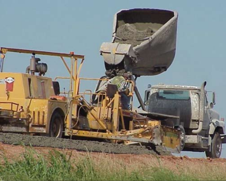
CIMARRON TURNPIKE - PAVEMENT REHABILITATION
