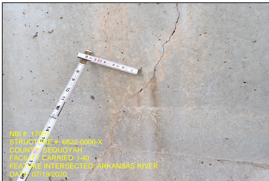
Photo 12 – Pier 4, typical cracking
