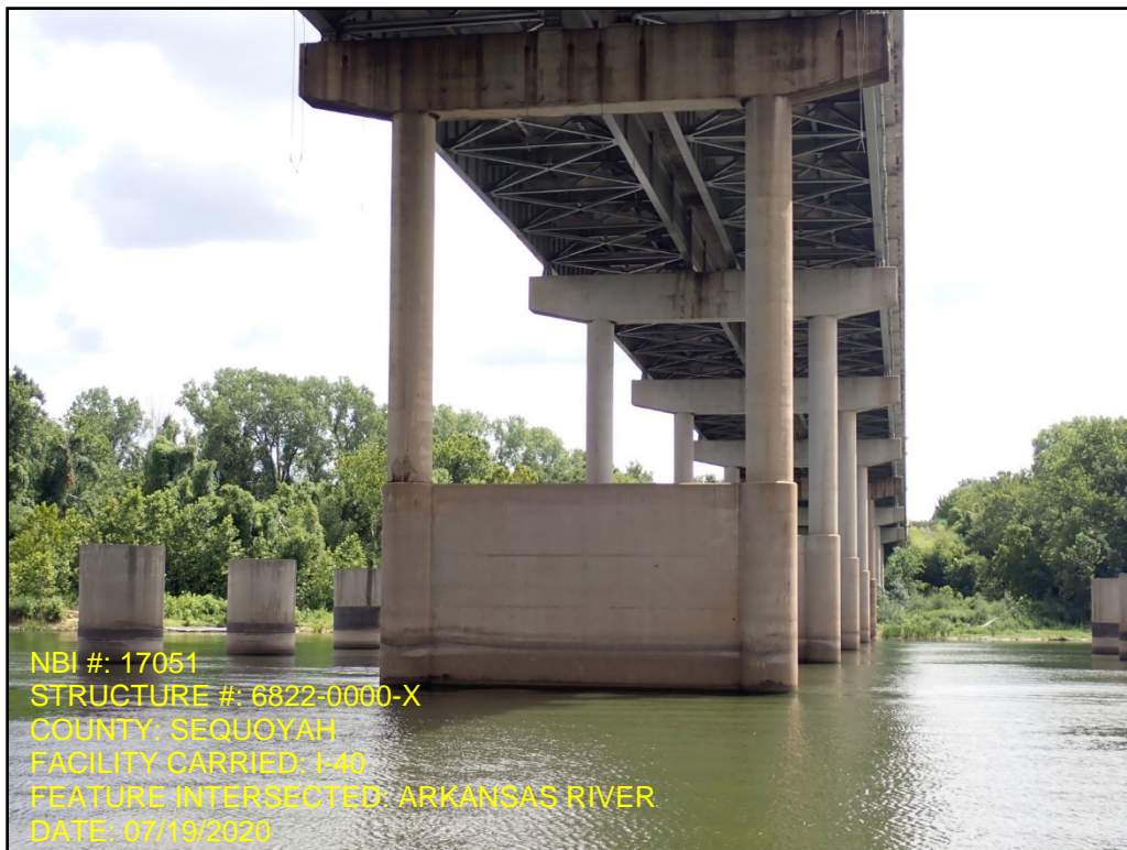
Photo 6 – Pier 6, typical configuration for Piers 6-10
