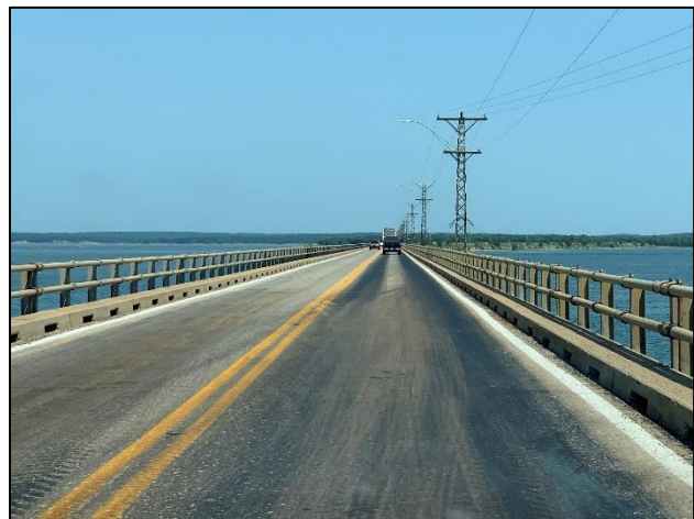
Figure 2: Roosevelt Bridge Narrow Deck Width
