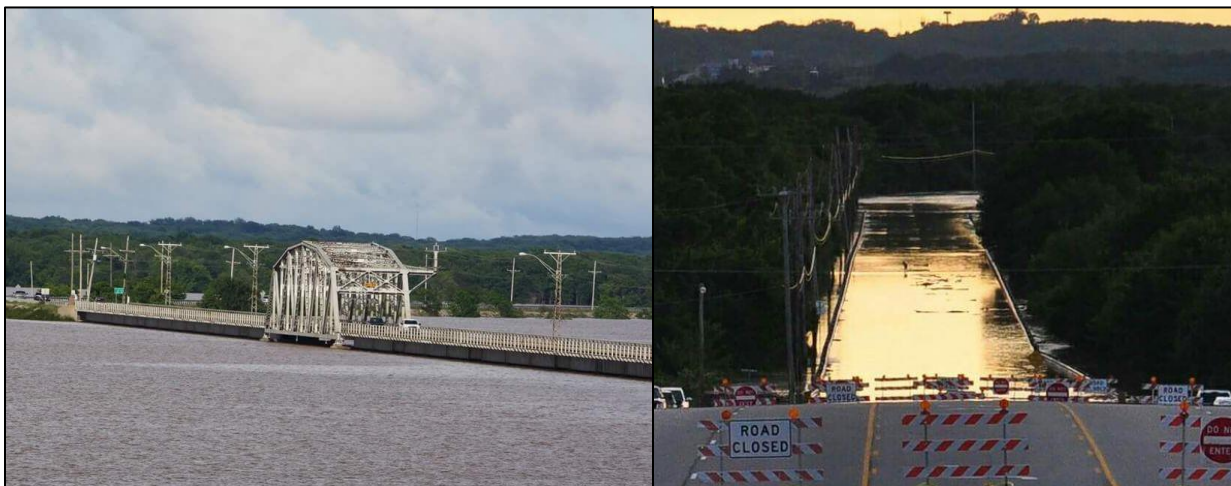
Figure 5: Roosevelt Bridge Flooding, 2015
