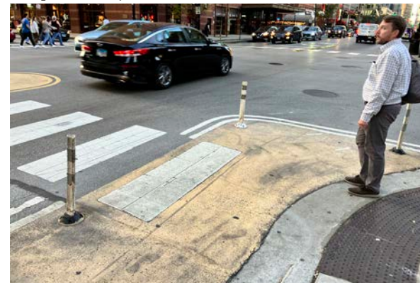
Example of an intersection narrowing using paint and flexible bollards.
