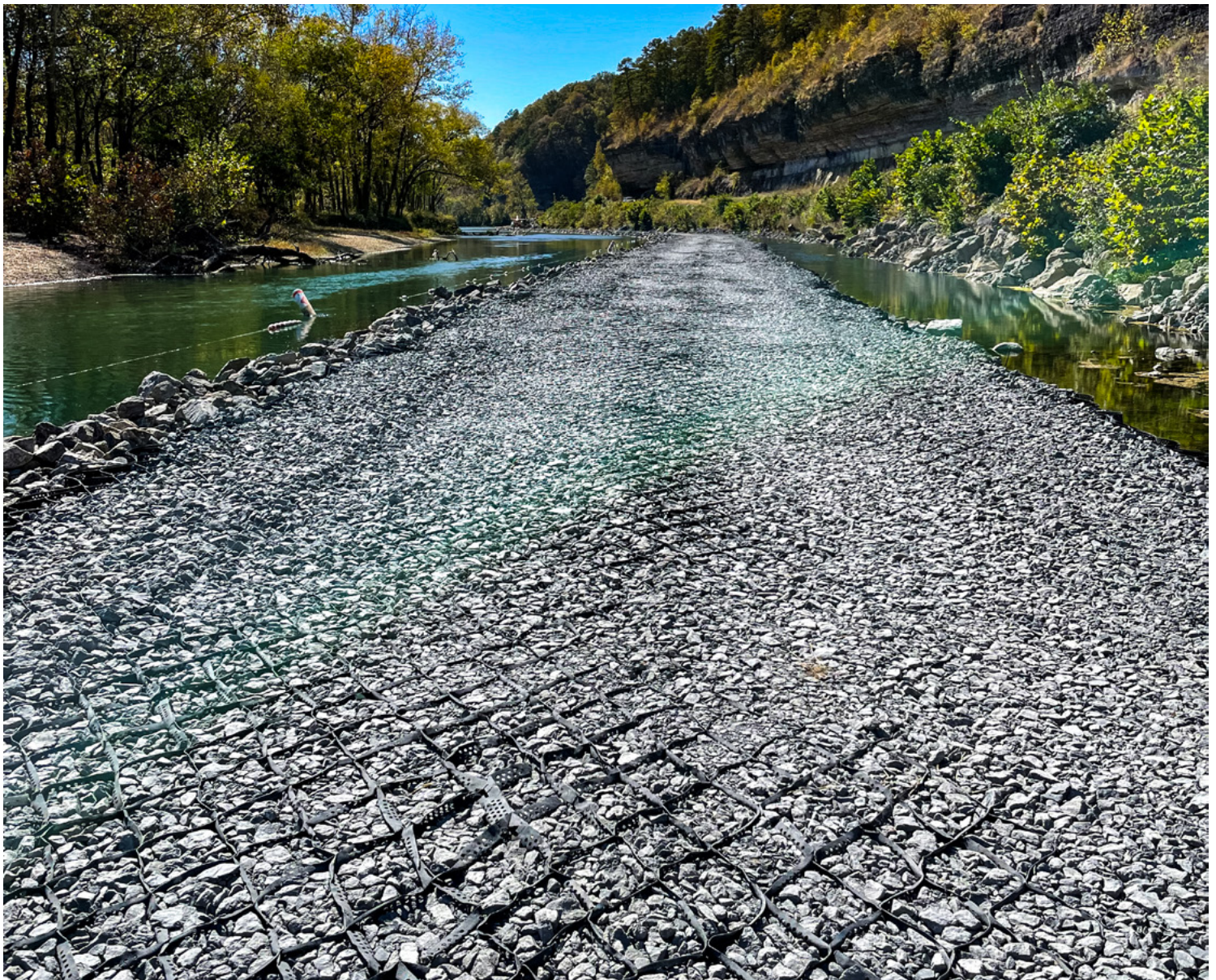
The retaining wall in the Illinois River was constructed to combat erosive effects on its slopes.
