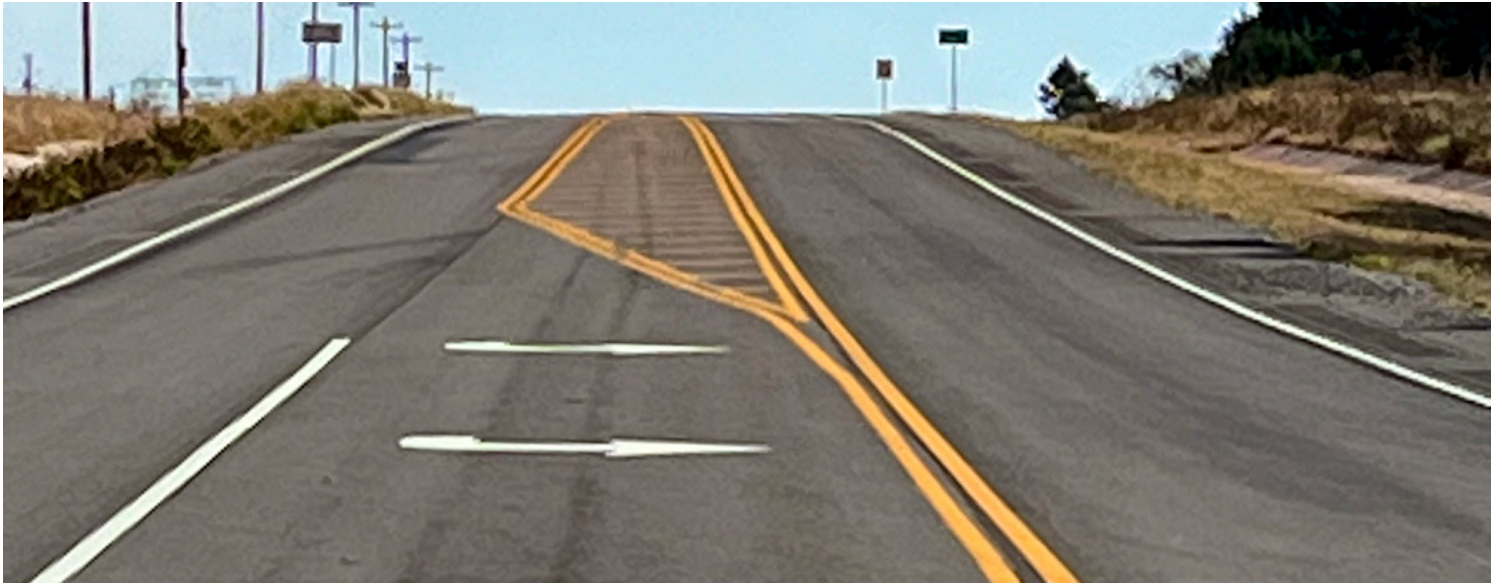
Facing East: A hill on SH-39 creates limited visibility for drivers approaching the SH-102 junction from the east, which is why the new left turn lane and shoulders at this location are essential for driver safety.
