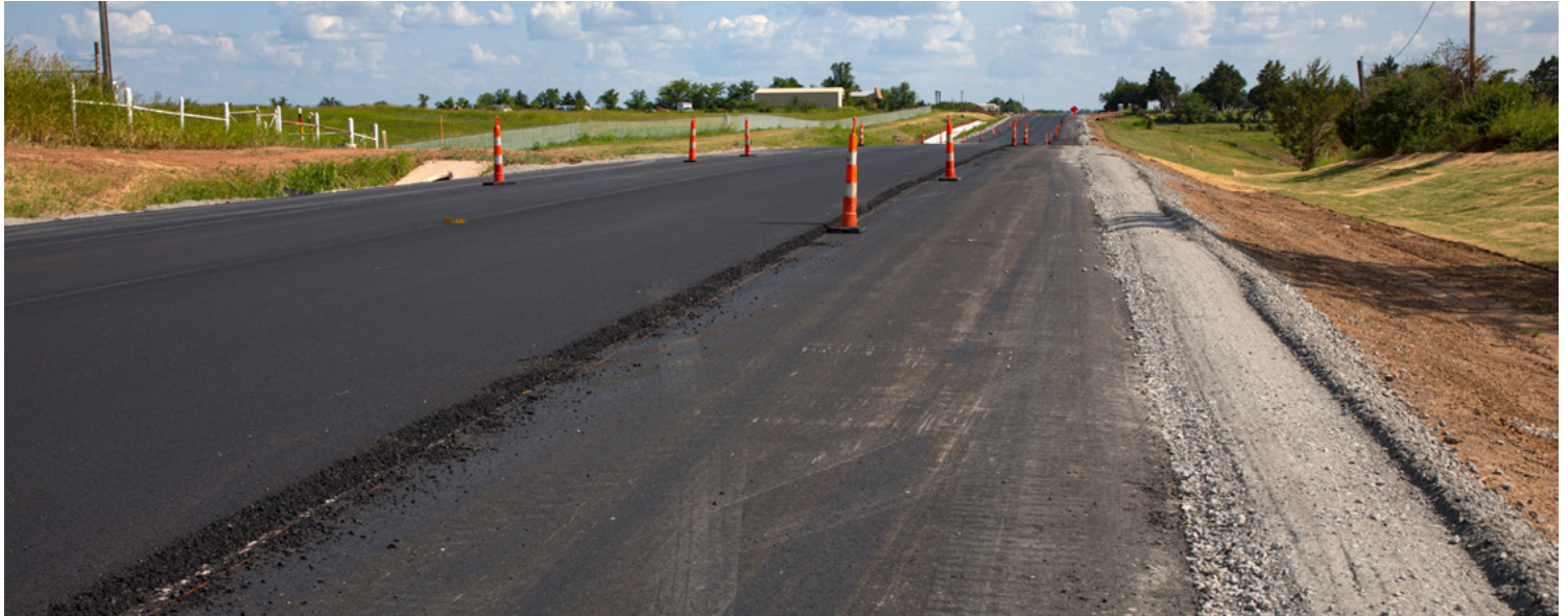
Shoulder construction in rural Oklahoma.
