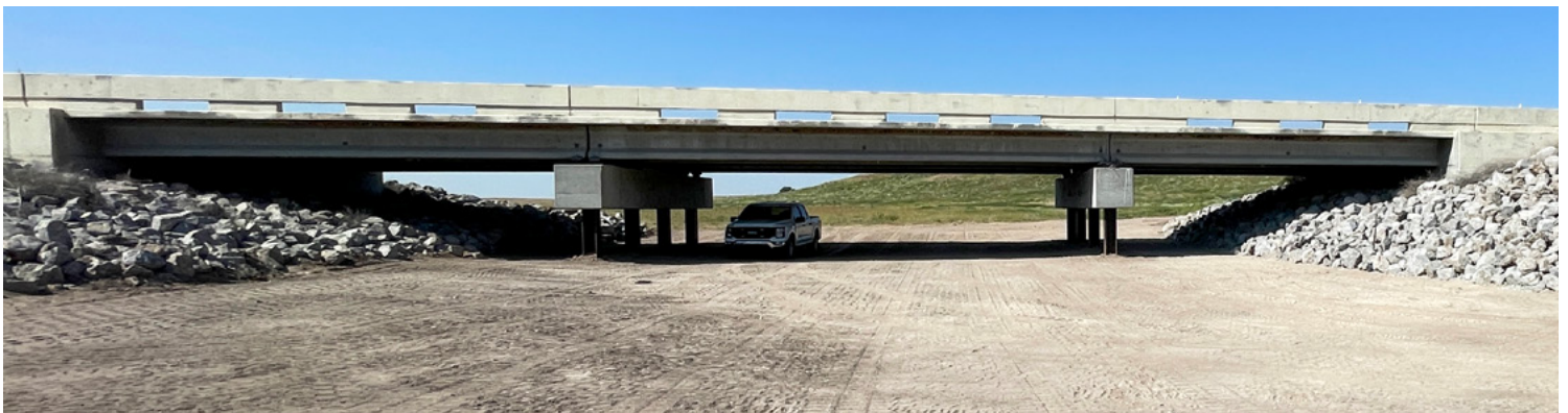
Filling the scour hole took three-hundred cubic yards of material to achieve. District 6’s crews completed this job in less than one month.
