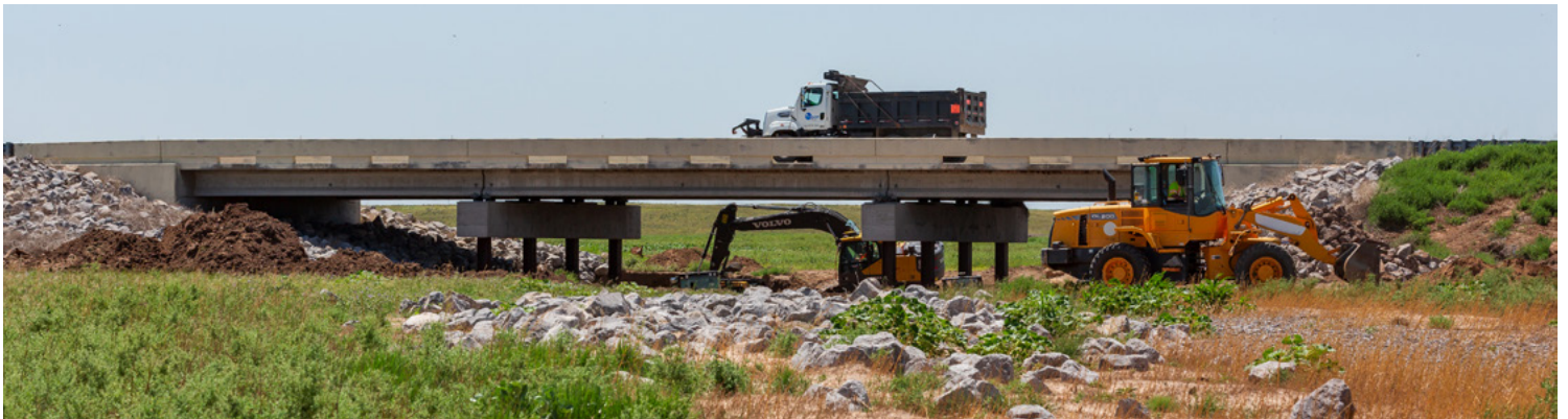
District 6’s maintenance crews work to fill and compact the scour hole with materials.
