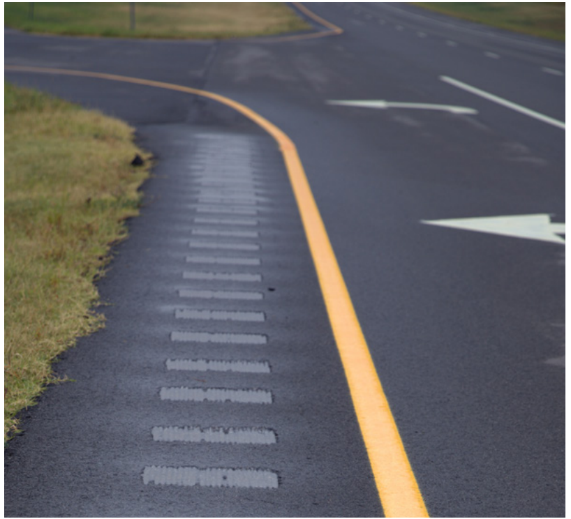
A rumble strip's vibration and noise is designed to alert drivers that their vehicle is leaving the travel lane.
