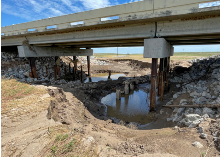
Under the Three Seeds Draw Creek bridge, water fills the 12-foot-deep scour hole.
