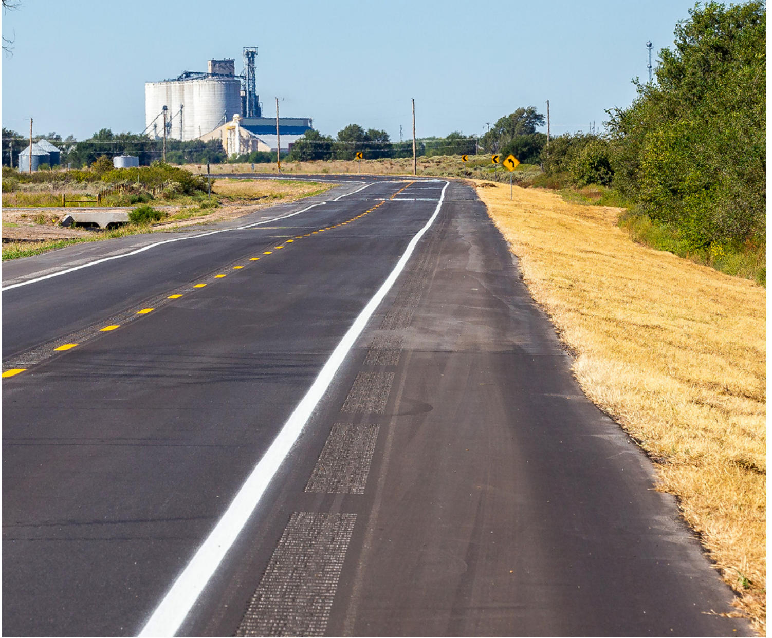
The SH-15 project between Woodward and Shattuck included a crown shift (or tilt in the road) to help travelers maintain control while driving near the railroad, which is located to the right of the pictured view, out of frame.
