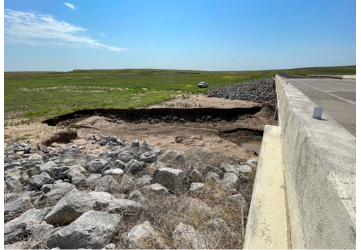
Bridge scour happens when underwater sediment is washed out from under a bridge’s foundation.
