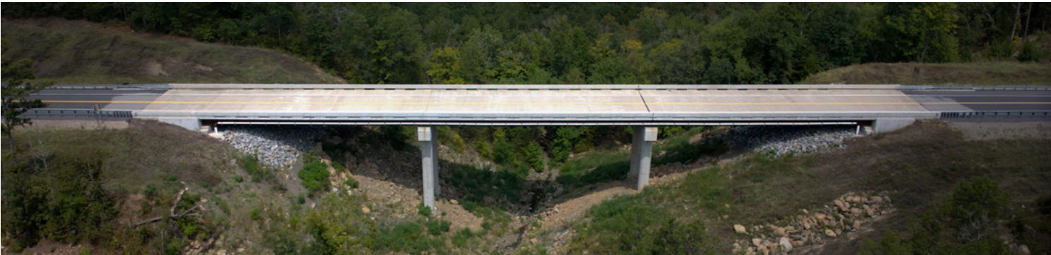
The new bridge over Sulphur Canyon on US-271 was a critical replacement due to the condition of the previous bridge, which was structurally deficient and functionally obsolete.
