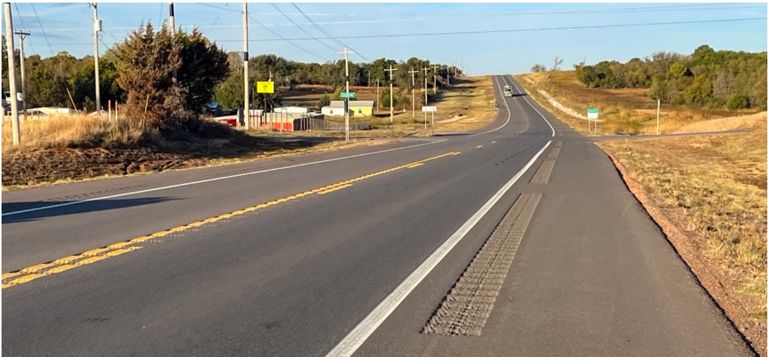
Facing West: New shoulders on SH-39 at the Grady and McClain County line.
