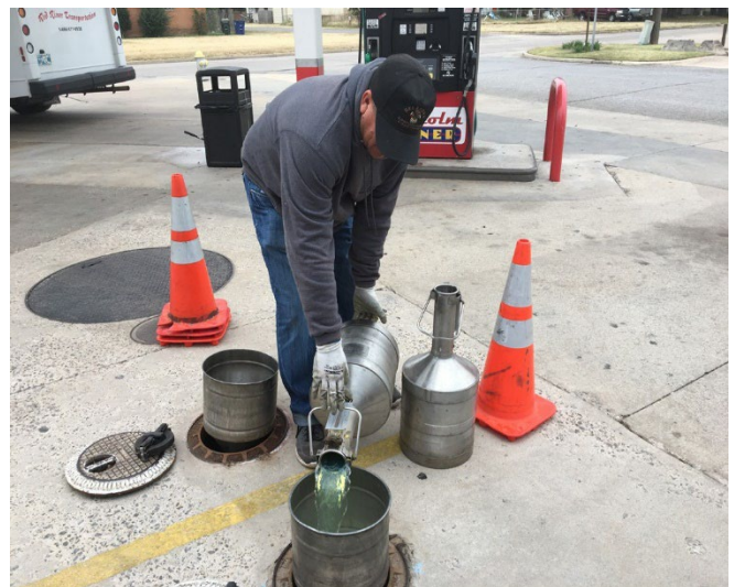
Figure 4 Fuel Inspection Supervisor Ty Massey demonstrates how to return fuel to an underground storage tank after fuel has been tested
