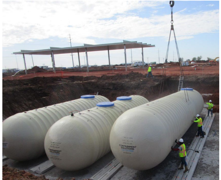
Figure 5 Installing Underground Storage Tanks at Loves on I-40 and Post Road in El Reno
