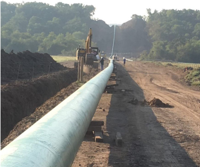
Figure 7 Mitch Skinner of The Pipeline Safety Department inspecting a Kiowa Power Partners, LLC construction project. The five-mile 24-inch pipeline will be providing fuel to the Kiamichi Power plant in Pittsburg County
