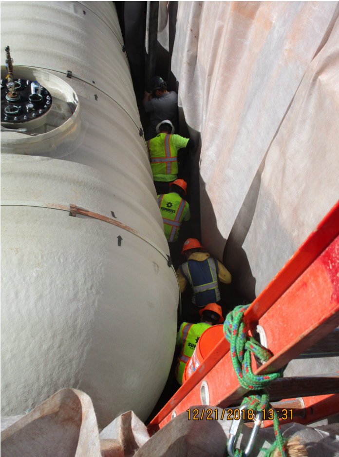
Above: Workers install gravel bedding at the bottom of an underground storage tank at a Costco fueling station in Oklahoma City as the facility was under construction. Inspection and Enforcement Department staff oversee installations.
