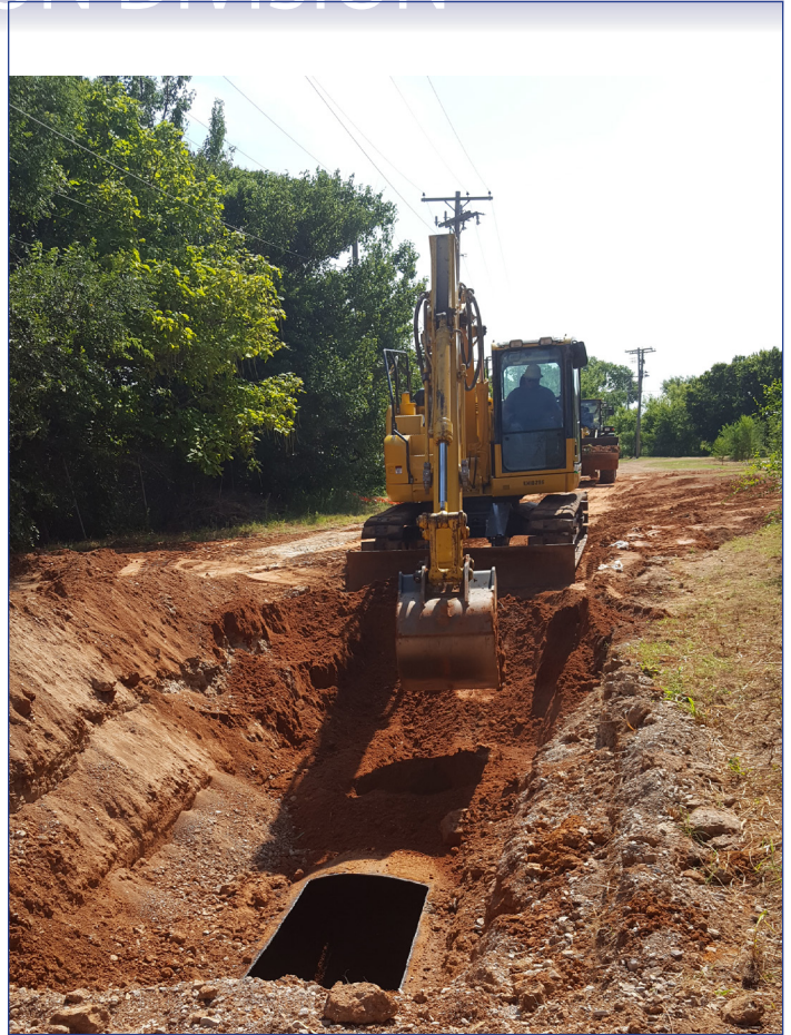
Above: A worker operates a backhoe to excavate an underground storage tank as part of a Brownfields cleanup project.
