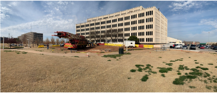
Above: A drilling rig lowers its mast after plugging a purging gas well in front of the Oklahoma Tax Commission in March, 2019. OGCD staff oversaw the plugging process.
