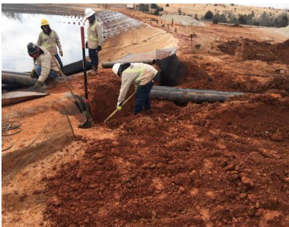
Above: Construction contractors work at a water reuse pit.
