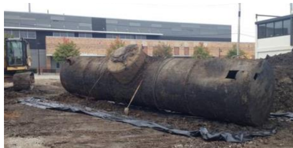
Above: The Gates Hardware building in Tulsa had an old railcar that was used for underground petroleum storage. Brownfields funding helped remove the tank so the company could expand its parking lot.
