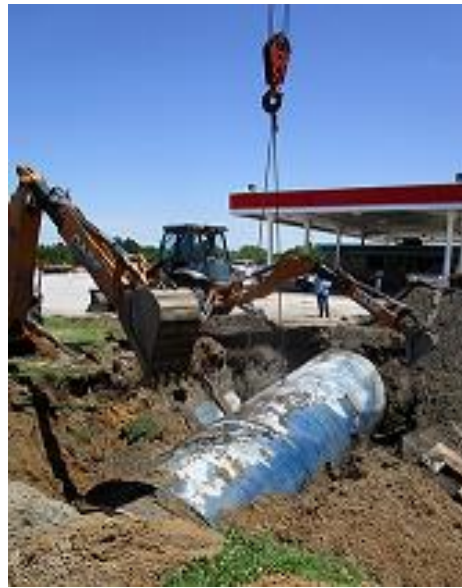
Above: Until the mid-1980s, most storage tanks were made of bare steel, which is more likely to corrode over time and allow its contents to leak.
