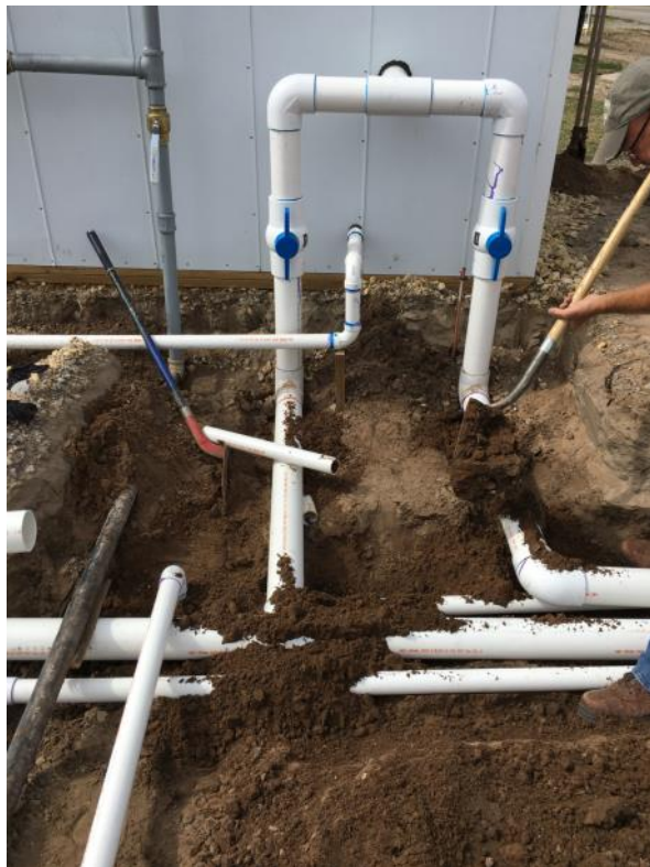
Above: A worker installs a vapor extraction system into the soil. The facility is an active gas station surrounded by commercial and residential water supply wells.
