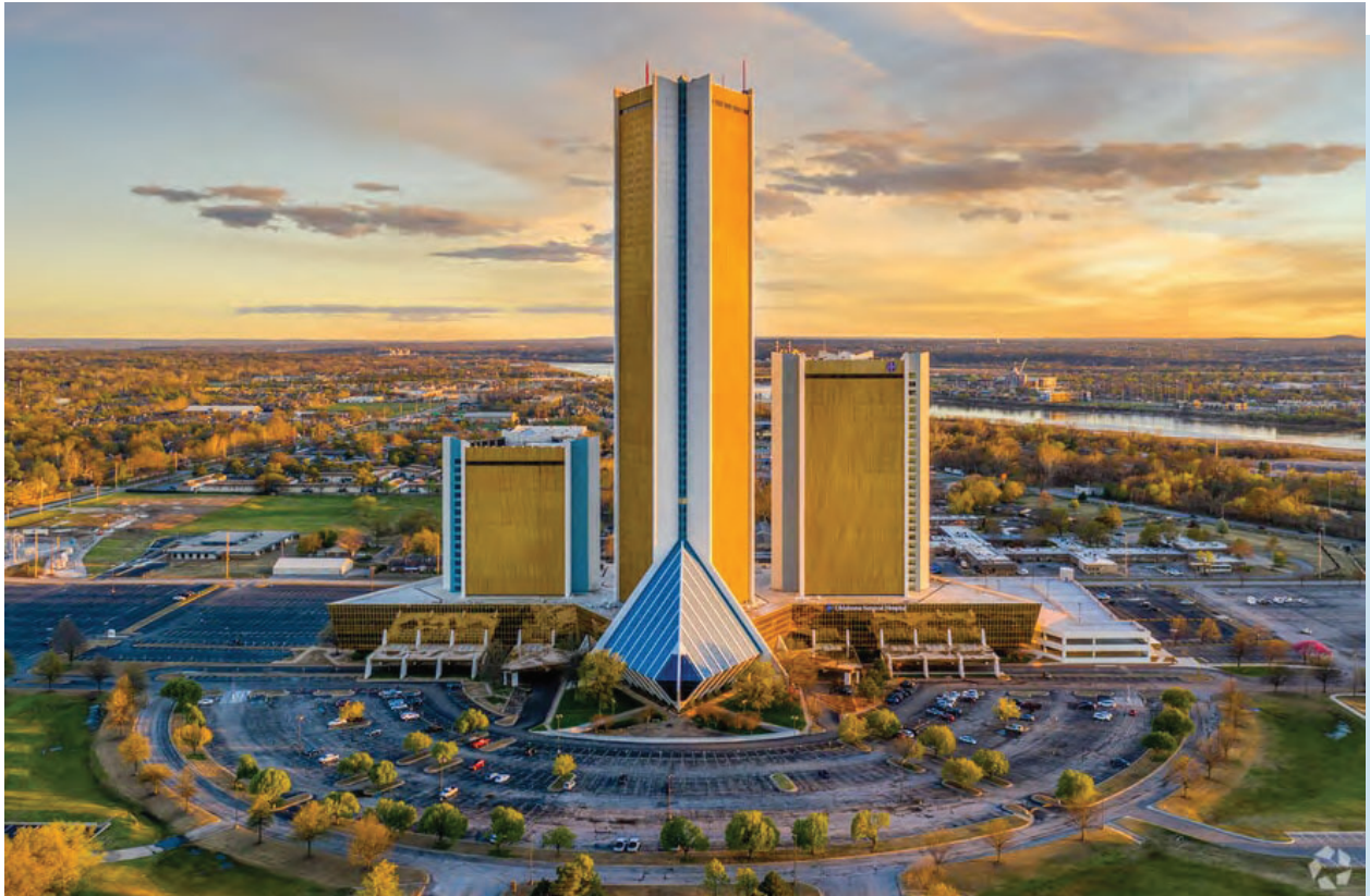
Figure 3 - The roofs of office buildings, such as CityPlex Towers in Tulsa, may host vertiports.
