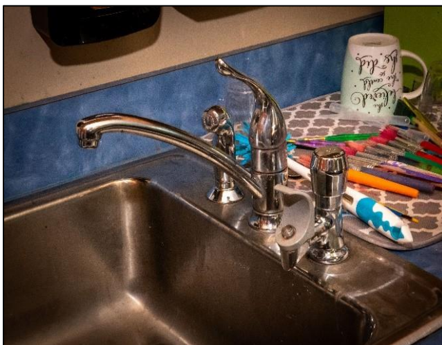
The image above is of a Classroom Faucet (CF) and Drinking Water Fountain (DW) that were sampled at a school. There were multiple schools with two (2) fixtures on each sink. These are often found in schools built prior to 1980.
