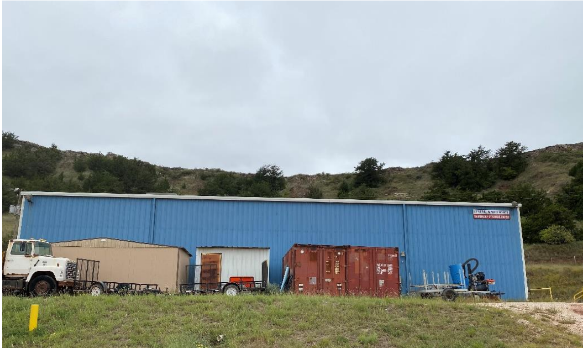
General Maintenance Building east side
