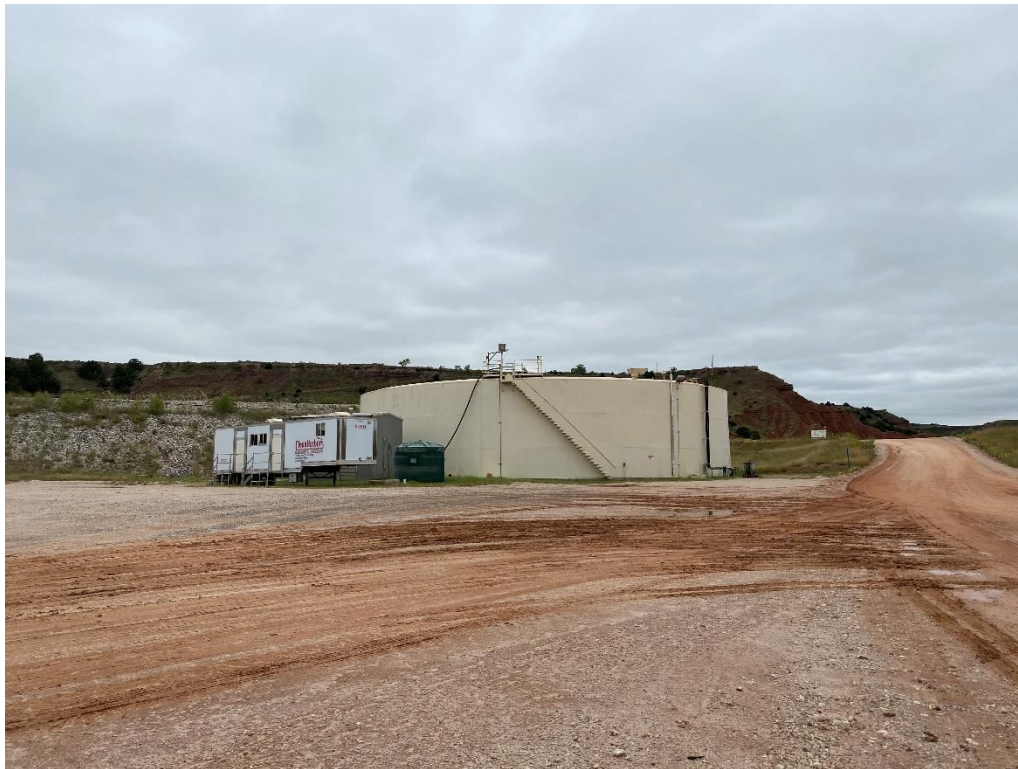
West facing T-6 Tank Storage Area
