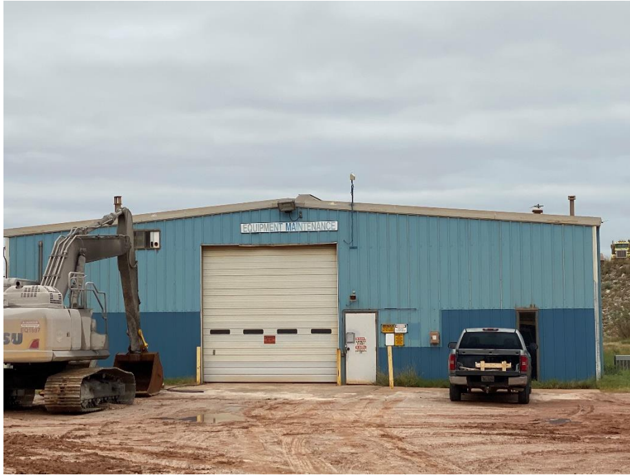
Equipment Maintenance Building
