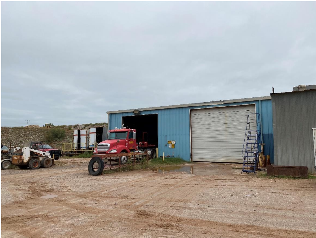
West side of Equipment Maintenance building
