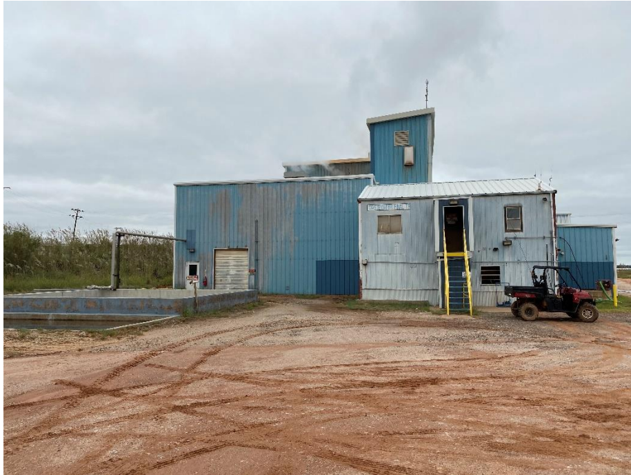
Wastewater Final Treatment Building
