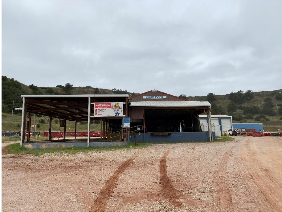
Drum Dock Building
