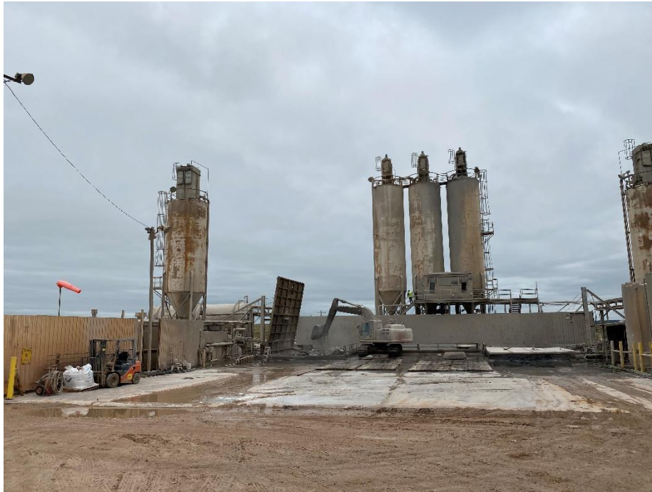
Stabilization Treatment Unit North Tank
