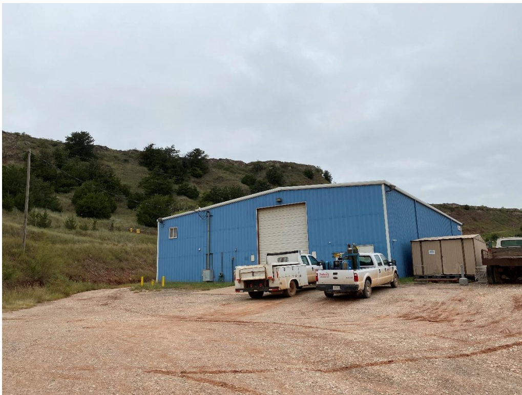
Entrance to General Maintenance Building
