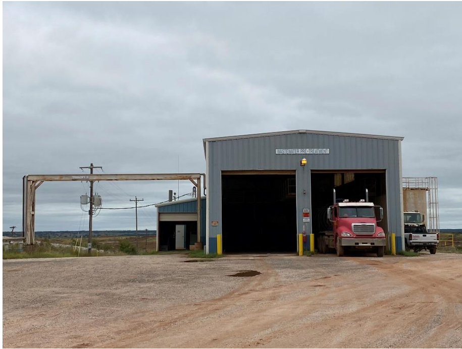
Wastewater Pre-Treatment Unloading Area
