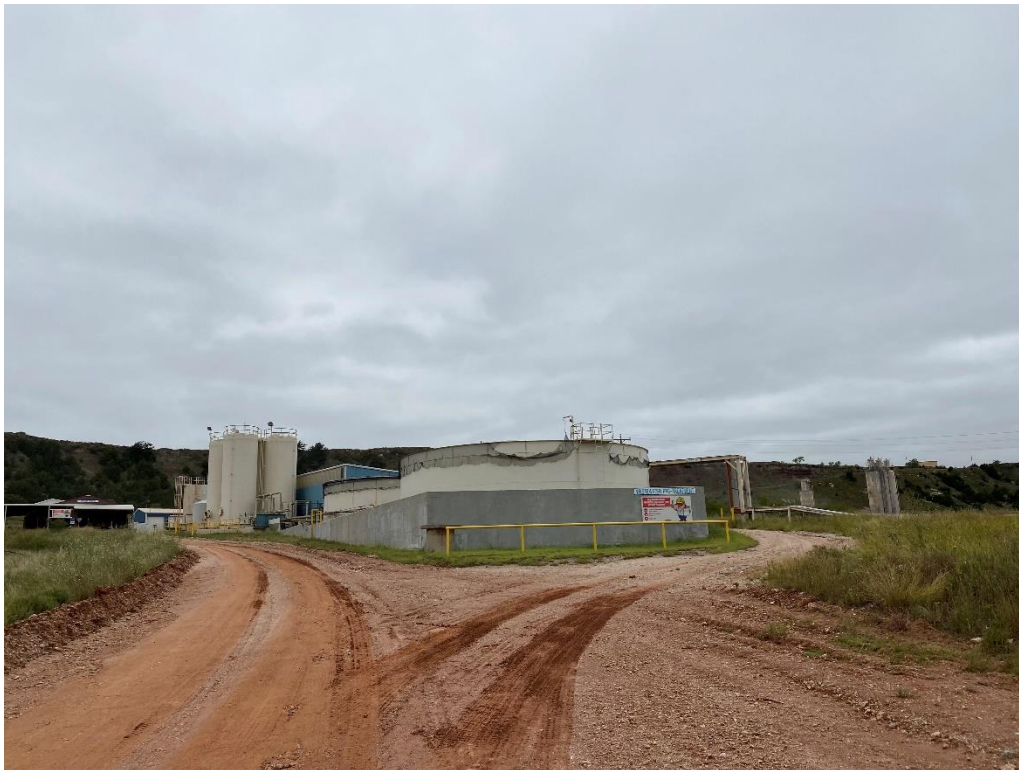
EF Tank Storage Area
