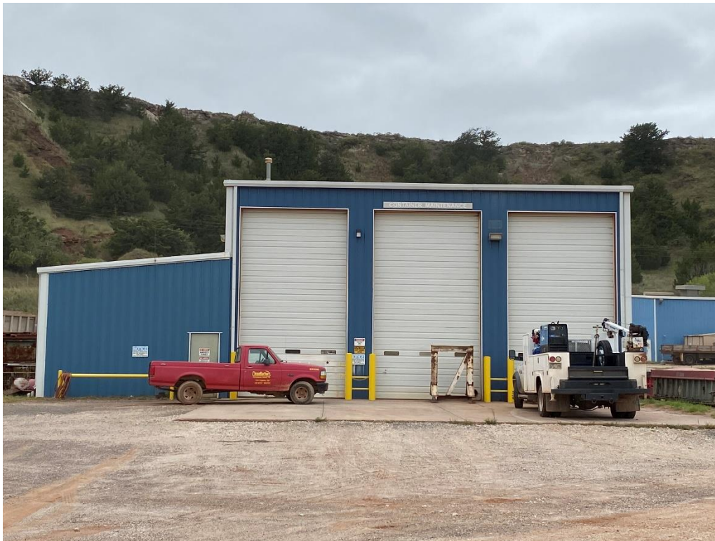
Container Maintenance Building
