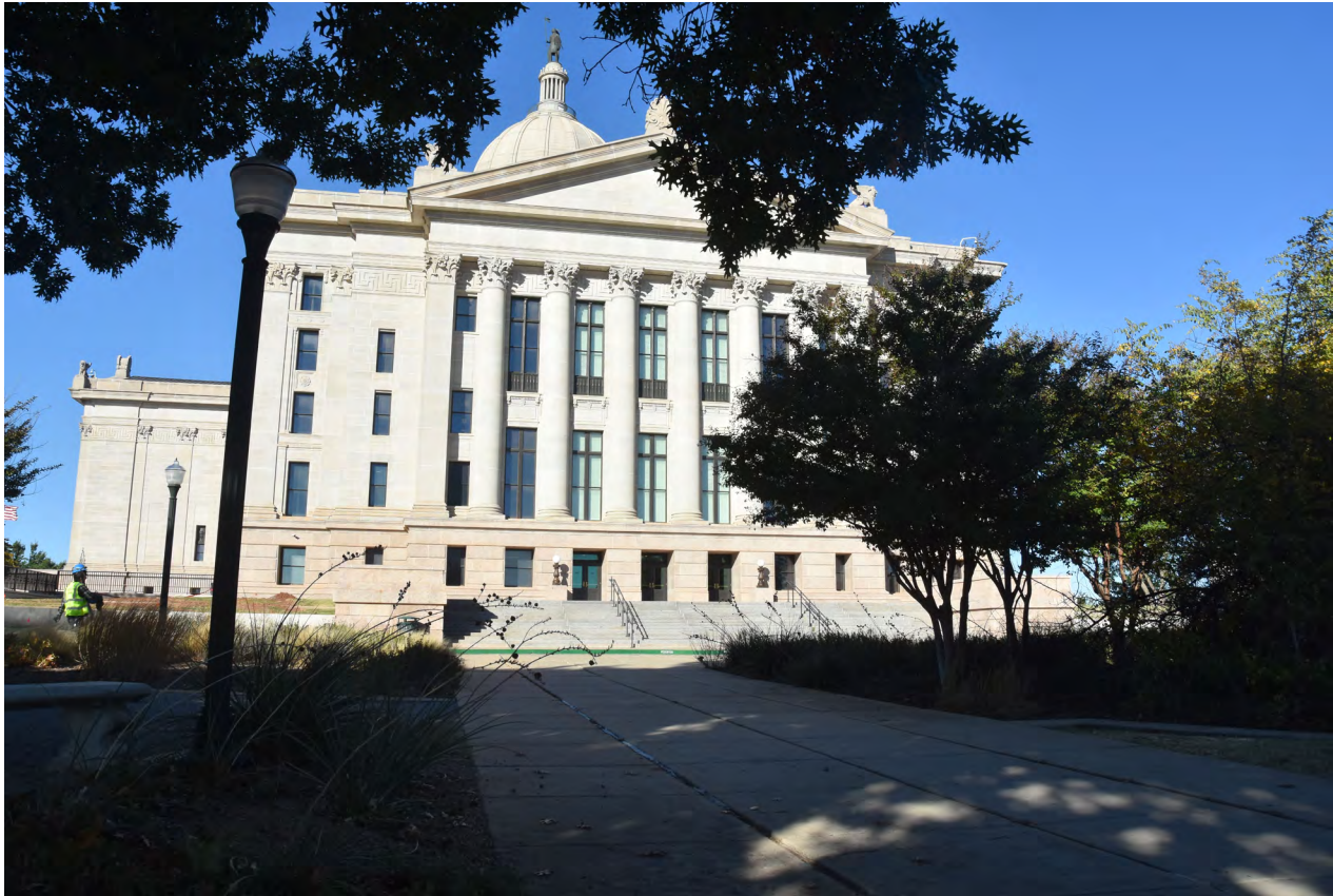
Top: The east side of the Capitol is shrouded in a cocoon of fabric in October 2017, while workers clean and repair the building’s exterior.
